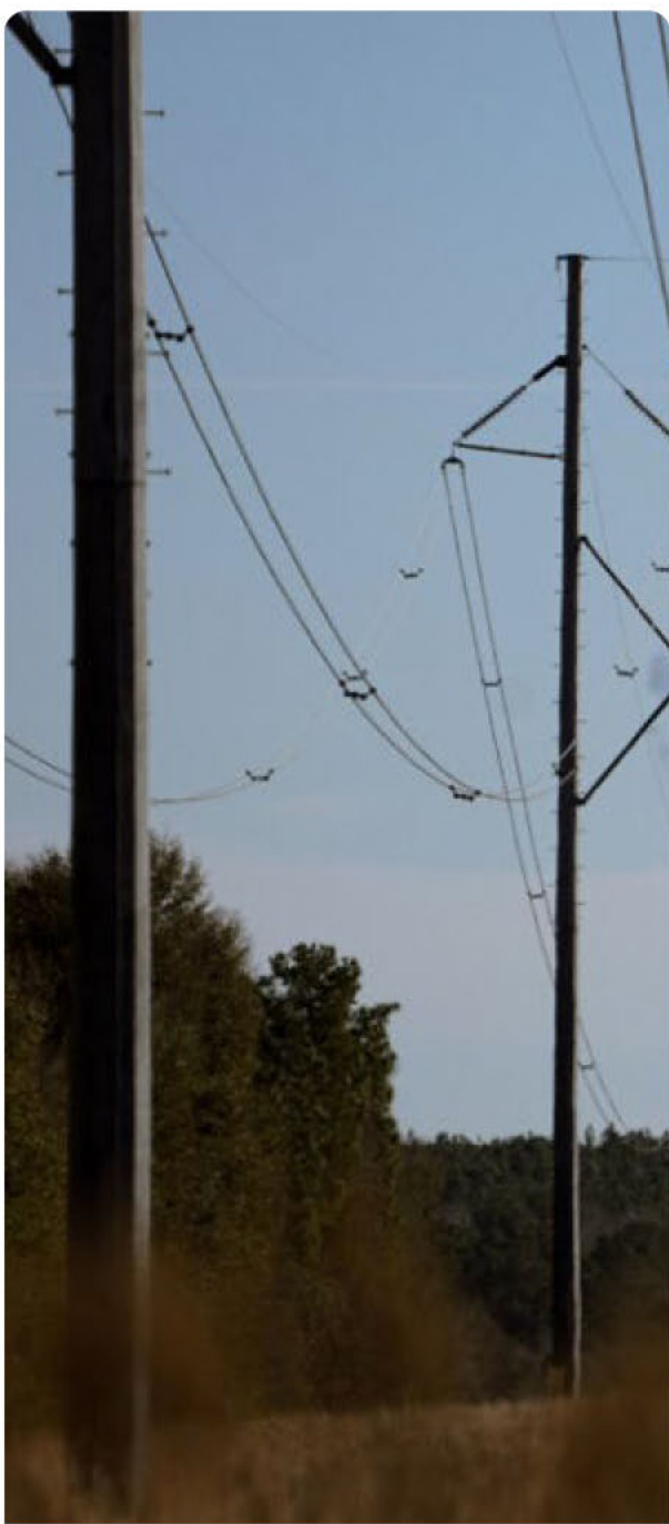
Georgia Utility Seeks Massive Grid Expansion To Feed Data Centers lists.theepochtimes.com
